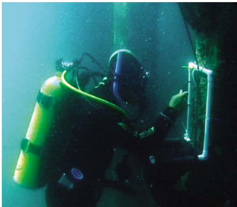
Figure 3: Diver sampling organisms on pier piles.
