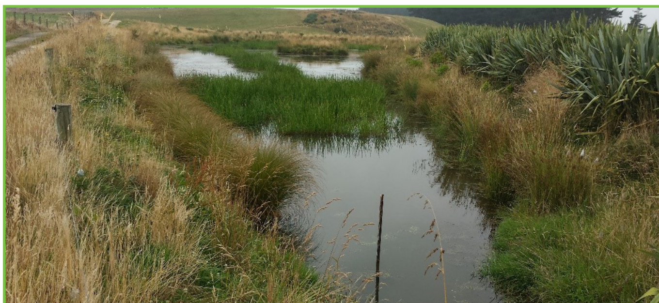
Wetland viewed from the inlet showing emergent beds of kuta and island in the background. Greater plant coverage particularly on the margins would improve the performance of this wetland.
