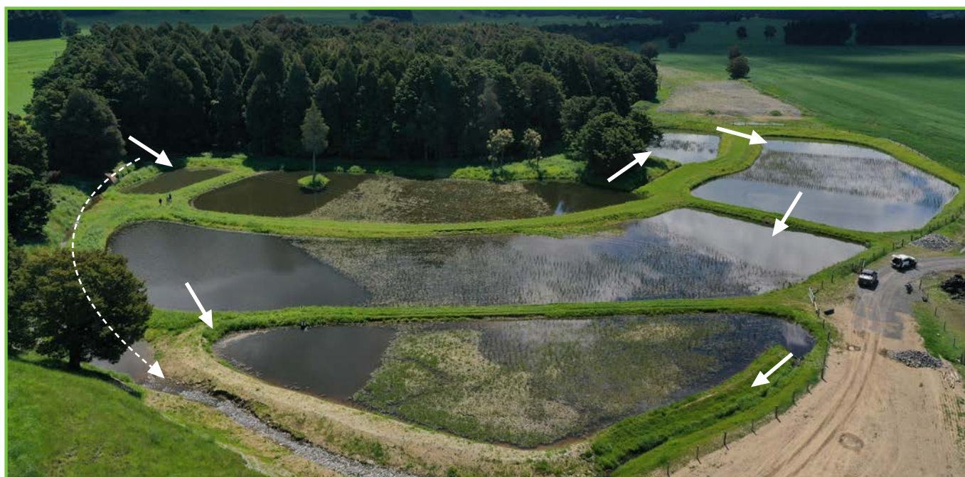
Establishing wetland plantings after six months growth. Arrows show flow path through the wetland cells. Flow enters in the top right from a stream that flows through the patch of native forest and from upwelling shallow groundwater. The dotted line shows high-level flow bypass channel.
