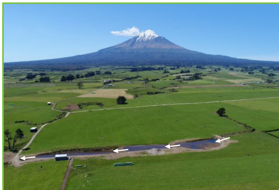
Newly constructed and planted wetland (left) showing direction of flow through initial deep sedimentation pond and subsequent two shallow elongated cells. Plant cover after one year shown on the right.
