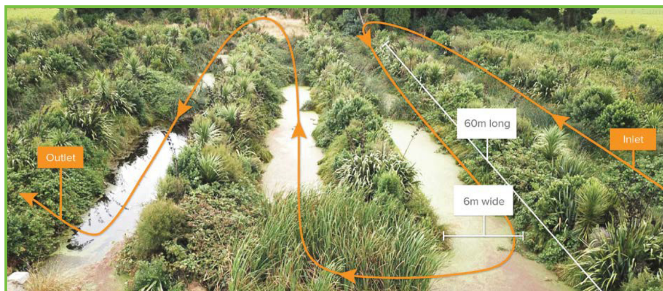
Photo shows serpentine flow-path through one section of the wetland. Shallower water depths would likely provide improved plant establishment and cover. Graphic courtesy of John-Paul Pratt (Groundtruth Ltd) and Neville Fisher (Kaiwaiwai Dairies).
