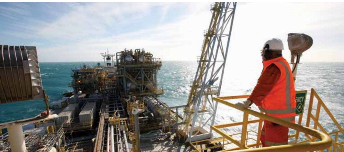
The Umuroa, an oil production and storage vessel, tends rigs in the Tui Area Development oil project, some 50 kilometres off the Taranaki coast. (NZ Oil & Gas)
