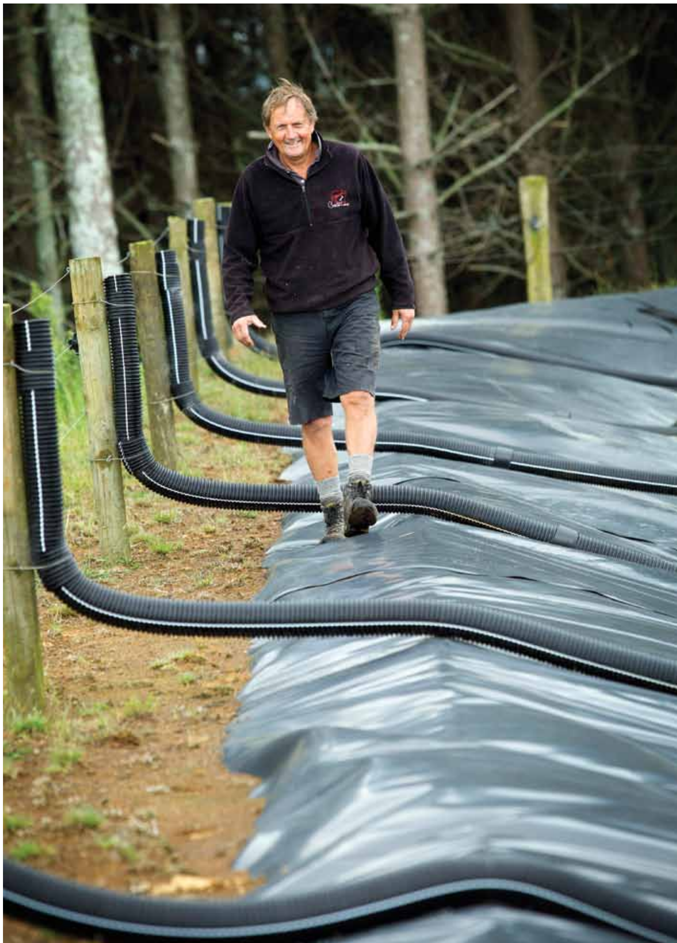
Taranaki pig farmer and biogas pioneer Steve Lepper. This anaerobic digester pond produces some 200m 3 of biogas a day. Scrubbed, compressed, and pumped to a generator, it now provides roughly half the piggery's daily electricity needs. (Geoff Osborne)
