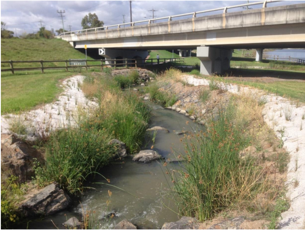
Figure 5-8: Example of a small low gradient nature-like rock ramp fishway on the Patterson River near Melbourne, Australia. Photo credit: Paul Franklin.
