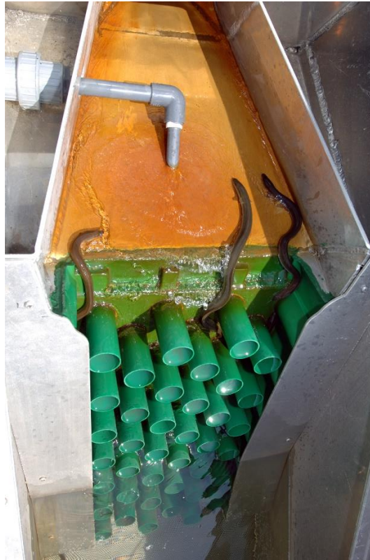
Figure 7-11: Milieu Inc. Eel ladder (for eels 150–750 mm) installed at the Moses-Saunders Dam. Photo credit: NY Power Authority.
