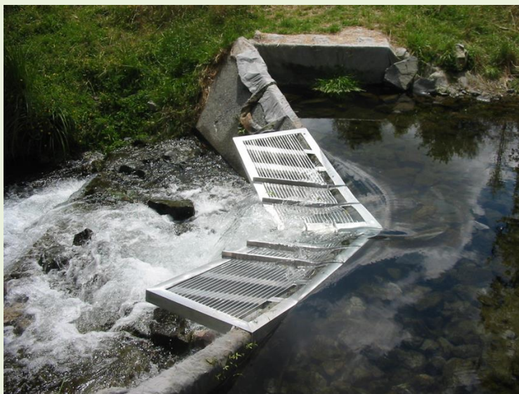
Figure 6-9: Trout barrier at Hamurana Springs. Photo credit: Andy Woolhouse.
