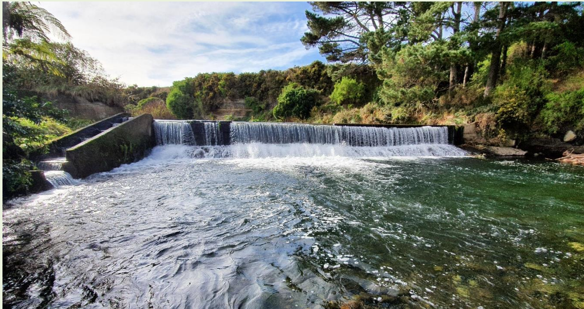
Figure 5-4: Kaūpokonui Stream weir prior to removal in 2021. Photo credit: Te Korowai o Ngāruahine.
