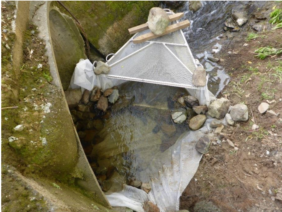
Figure 8-13: Whitebait trap installed at the culvert inlet in Kara Stream.
