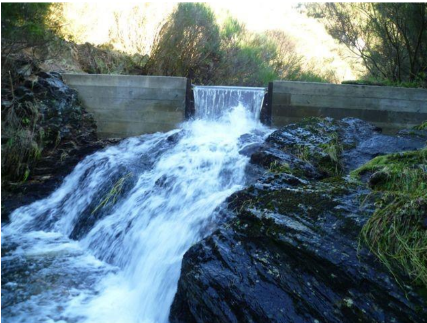
Figure 6-3: Akatore Creek barrier in Otago. A high head exclusion barrier installed onto a natural waterfall to protect Taieri flathead galaxias, after brown trout gained access upstream when conditions changed at the natural waterfall. Key features of the barrier are the height to prevent trout access, the overflow to minimise backwater creation and loss of non-migratory galaxiid habitat, and the wood boards to manage height and enable flushing if required. Photo credit: Sjaan Bowie.
