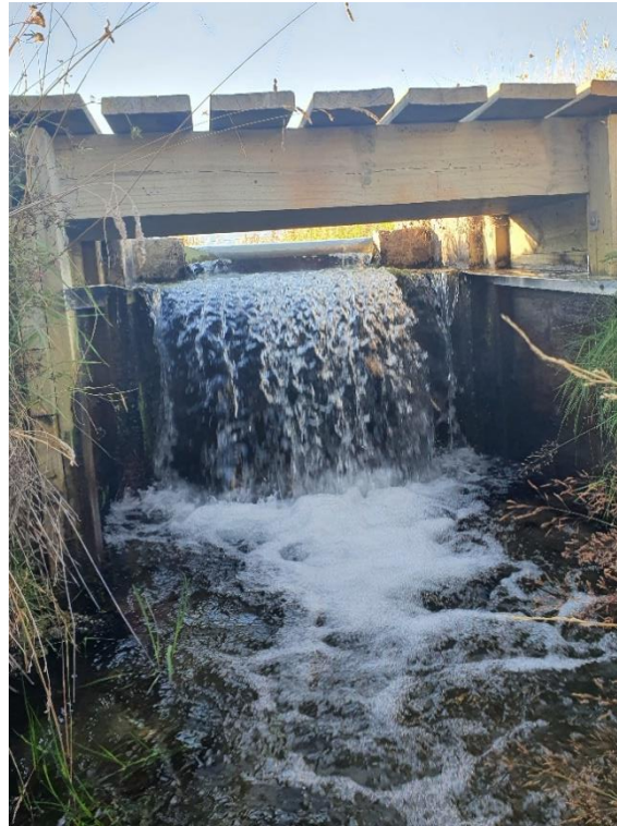
Figure 6-6: Exclusion barrier installed in an unnamed spring of the Fraser River. The objective was to prevent trout and kōaro accessing a key lowland longjaw galaxias and bignose galaxias stronghold in the MacKenzie Basin, Canterbury. Key features of the barrier were the height (0.83 m) and shallow downstream zone (concrete splash pad) to prevent trout access, the metal lip (300 mm wide at barrier face, 100 mm on concrete sides, 150 mm on wooden sides of bridge) to prevent kōaro passage (seems to be unsuccessful), and the wooden drop logs to allow for flushing of flows and maintenance of flows and habitat upstream. Photo credit: Sjaan Bowie (DOC).
