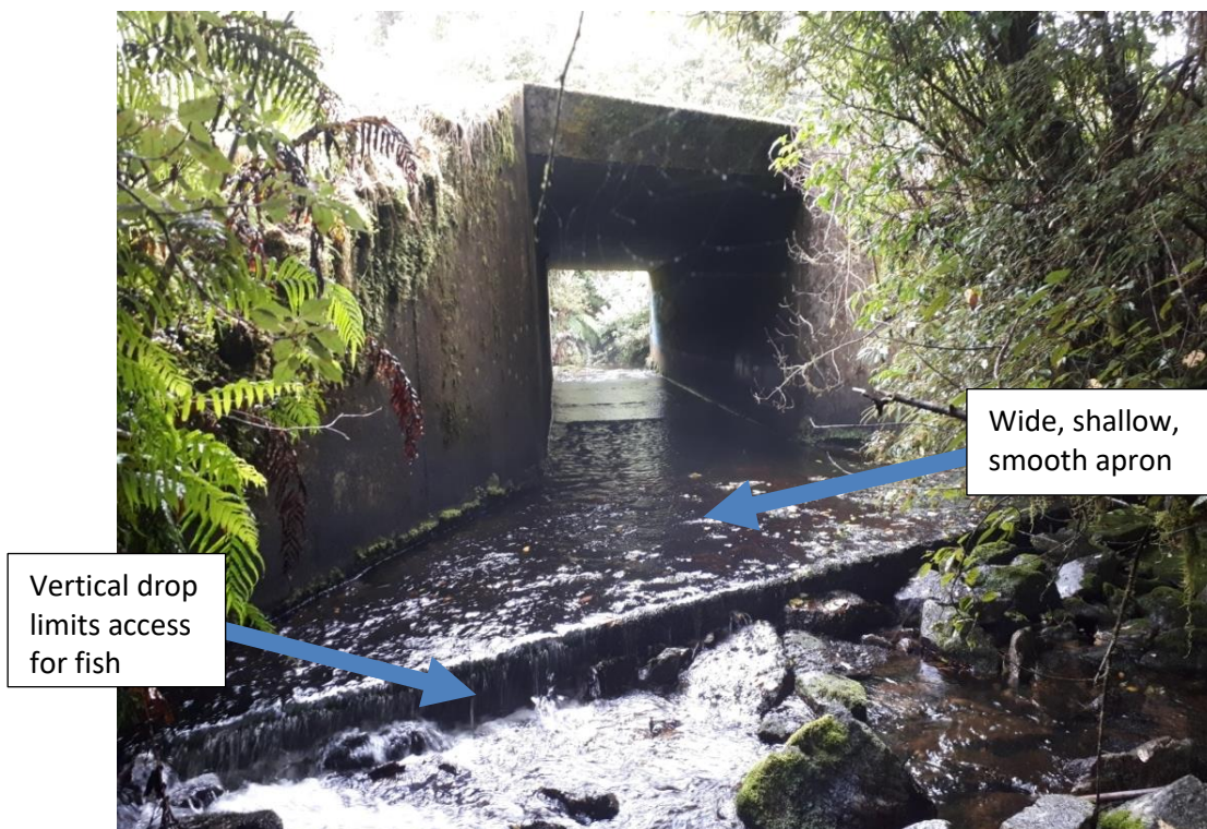
Figure B-17: Fish movements will be impeded by the fall at the downstream end of the apron and shallow water on the apron. Photo credit: Sam Ammon.
