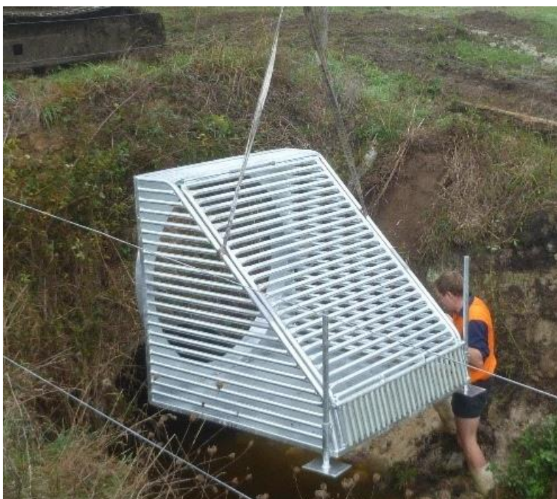
Figure 6-12: One-way gate structure prior to installation showing screen that can be lifted for inspection and clearing of debris. Photo credit: Adam Daniel.
