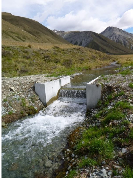
Figure 6-4: High head exclusion barrier installed in Fork Stream, Canterbury. The barrier was built to prevent trout accessing a key non-migratory galaxias stronghold in Fork Stream, Upper Waitaki River, Canterbury. Key features of the barrier were the height and downstream shallow zone (concrete splash pad) to prevent trout access, and the adjustable boards that can be slotted in and out to flush the habitat, minimise backwater and increase height if needed. Photo credit: Sjaan Bowie.
