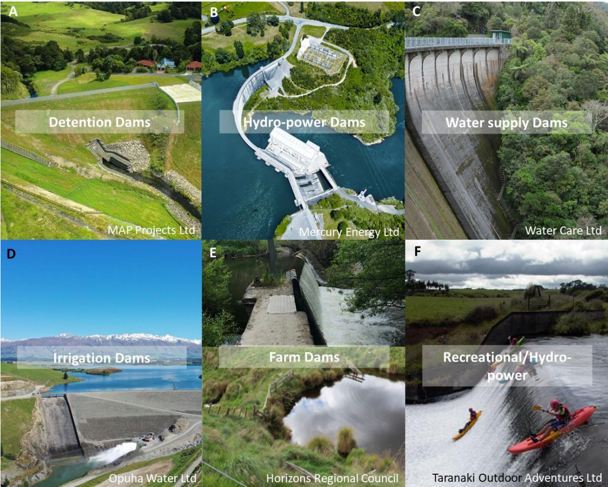
Figure 7-1: Examples of different dam types installed across New Zealand. A = Hopua Dam, Northland; B = Karāpiro Dam, Waikato; C = Upper Nihotupu Dam, Auckland; D = Opuha River Dam, Canterbury; E = Manawatū-Whanganui; Waingongoro River Dam, Taranaki.
