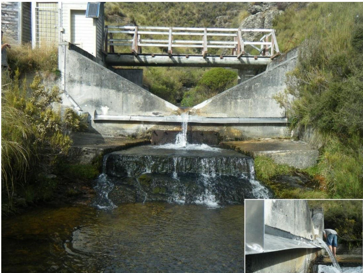
Figure 6-13: Full exclusion barrier installed in an un-named tributary of Upper Waipori River. The objective was to prevent trout and kōaro access to a key dusky galaxias stronghold in Otago. Inset shows a close-up view of the successful kōaro lip barrier. Key features of the barrier include the 175 mm depth aluminium sheet with 100 mm angle, sealed to the weir face with no gaps at a 120 degree downwards angle. Photo credit: Josh Tabak.
