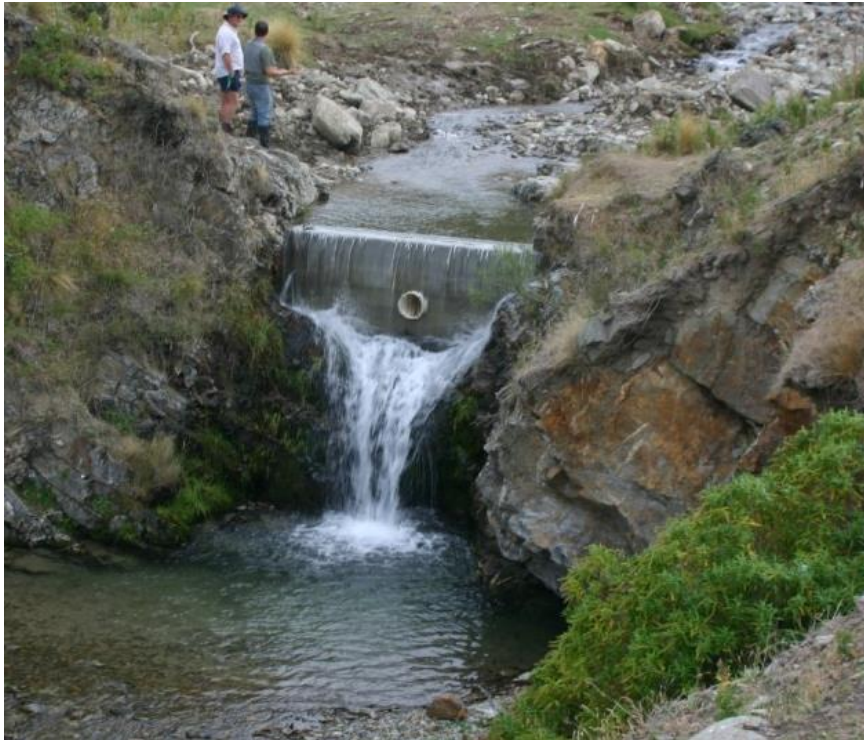
Figure 6-2: Swinburn Creek barrier in Otago. A high head exclusion barrier has been installed onto a natural waterfall to protect the Central Otago roundhead galaxias population, after brown trout gained access upstream when stream conditions changed. Key features of the barrier are the height to prevent trout access. Photo credit: Daniel Jack.
