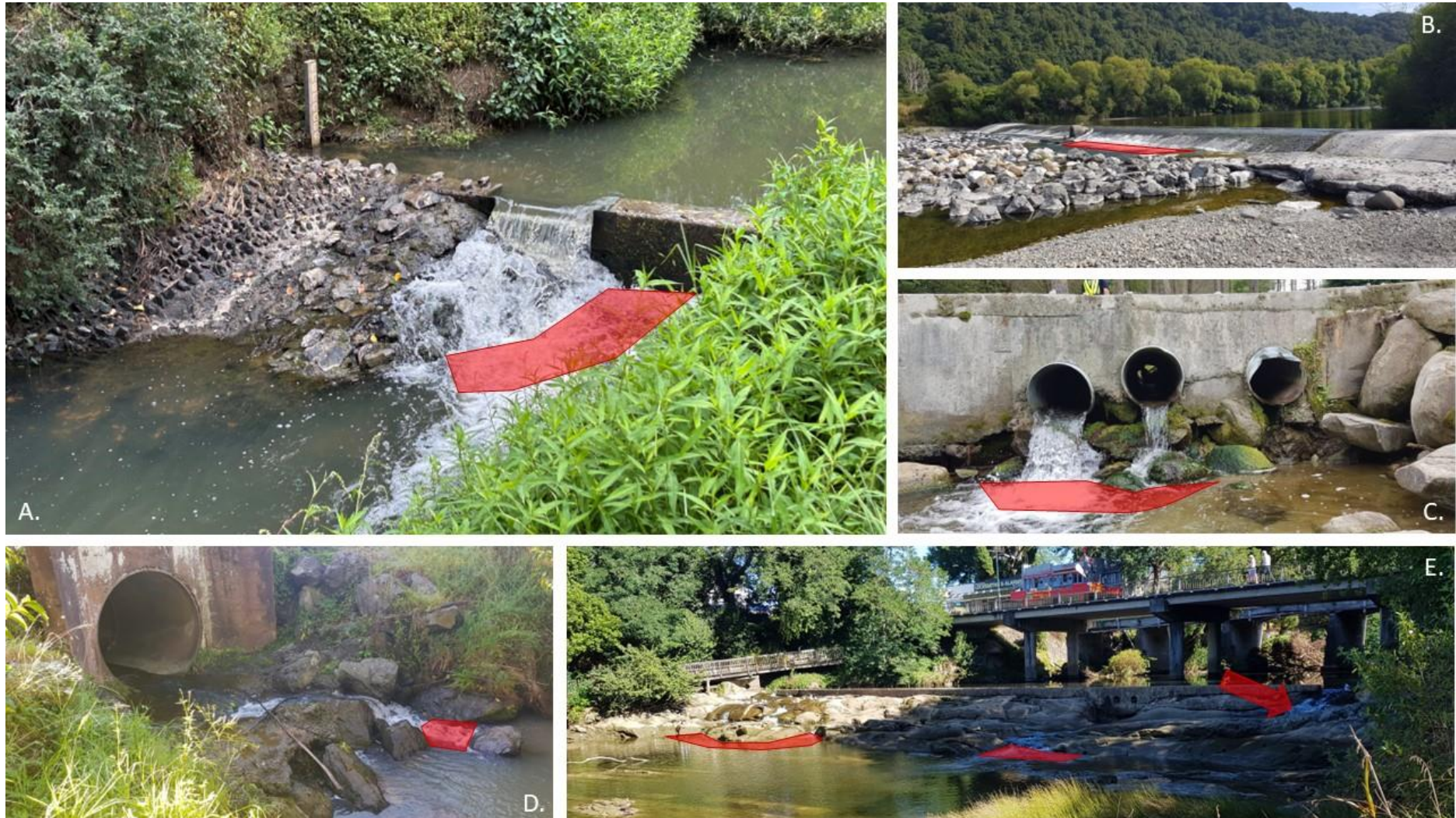
Figure 5-12: Locating the upstream limit of migration (area shaded in red). The upstream limit of migration is the furthest point upstream that fish can move to. The red areas show the upstream limit of location for structures A-E at the time the picture was taken. Note that site E is tidal and the upstream limit of migration moves from the shaded areas to the location indicated by the arrow at high tide.
