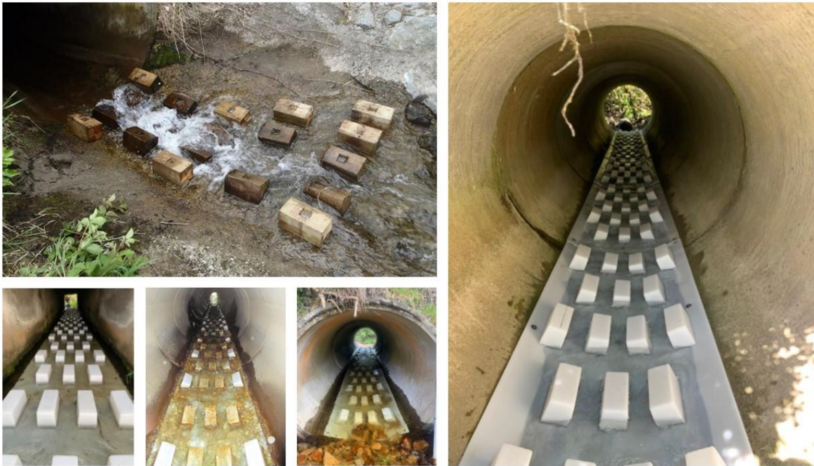
Figure J-2: Examples of spoiler baffles.
