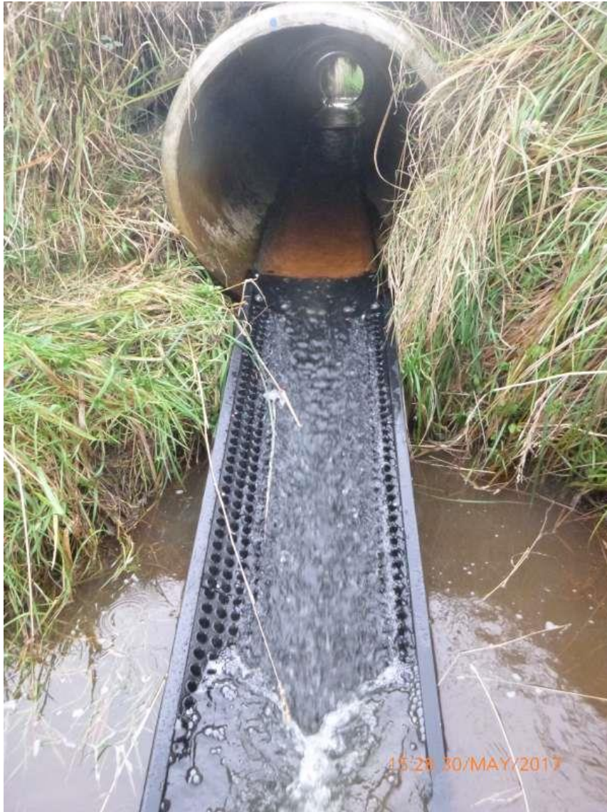
Figure 5-22: Example of an artificial fish ramp installed at a perched culvert in Southland containing the Miradrain™ substrate. Note that a shallow wetted margin is maintained on both sides of the ramp. Photo credit: James Dare.
