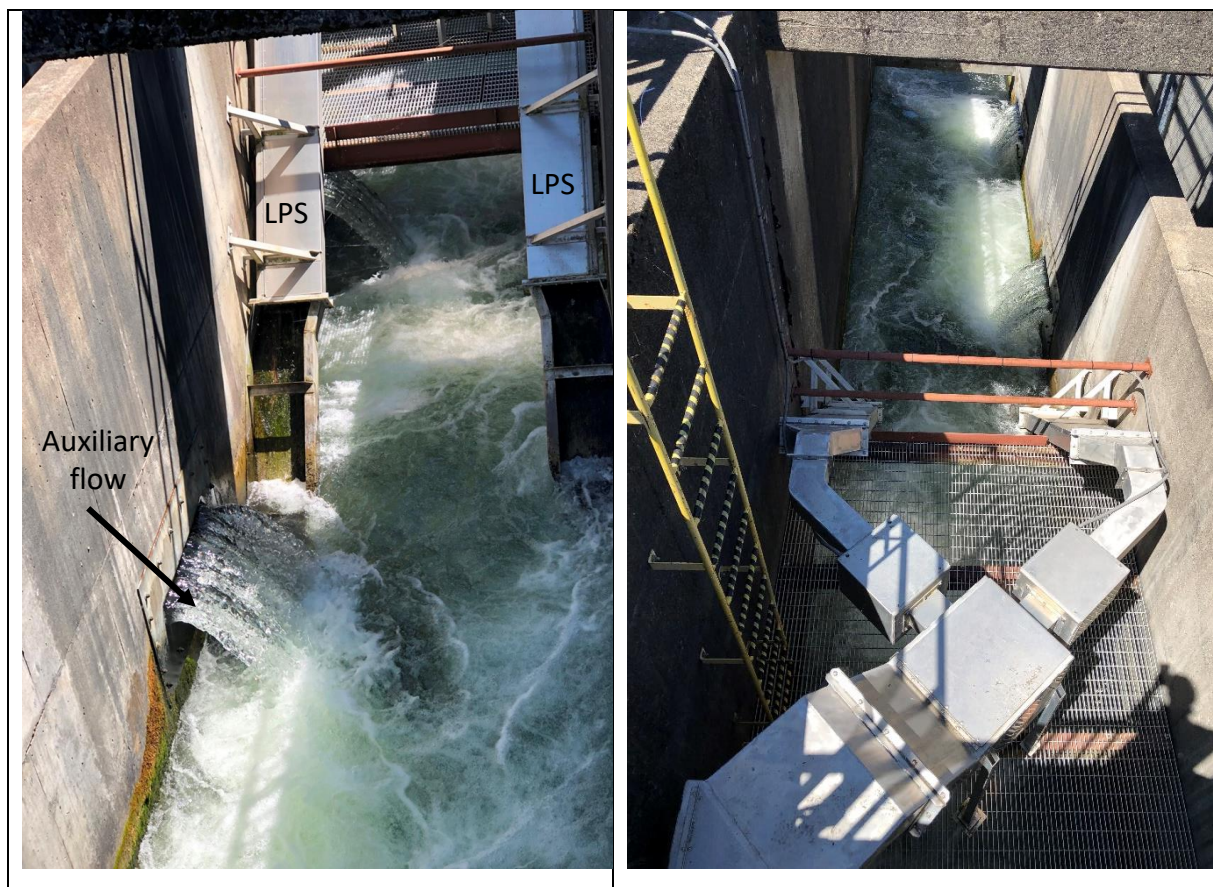
Figure 7-8: Lamprey passage structure (LPS) installed at Bonneville Dam, Columbia River, Oregon. Photo credit: Cindy Baker.
