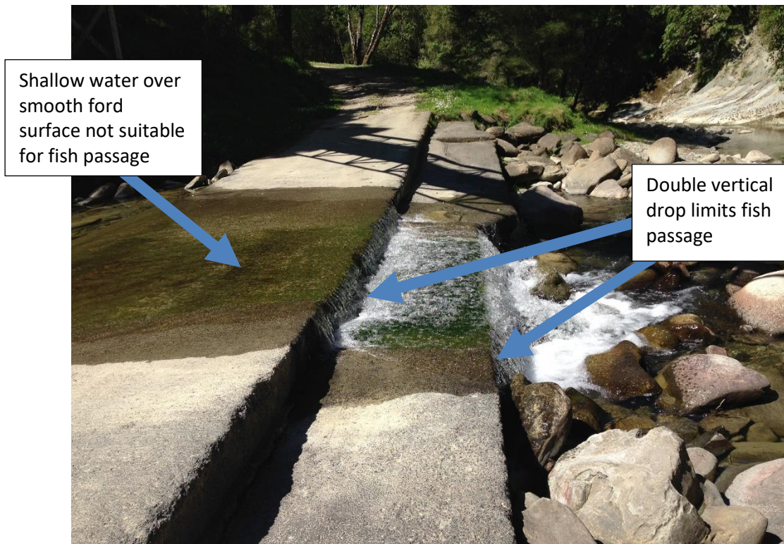
Figure B-20: Example of a ford from the Te Arai River. The fall height at the two steps on the downstream side of the ford makes a complete barrier to swimming fish species. Passage for climbing fish will be impeded by the sharp corners on the steps and shallow water across the ford, but some may access upstream habitats by taking advantage of the wetted margins to climb. Photo credit: Paul Franklin.
