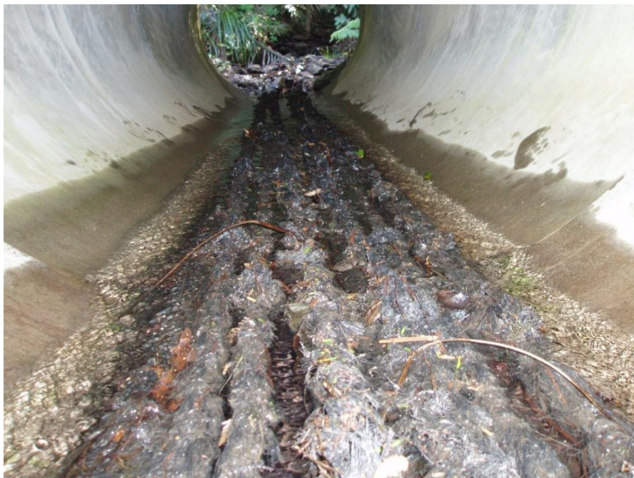
Figure 5-31: Example of good mussel spat rope installation showing fish 'swimming lanes' between ropes. Note that the number of ropes has been scaled up to match the size of the culvert. Photo credit: Bruno David.
