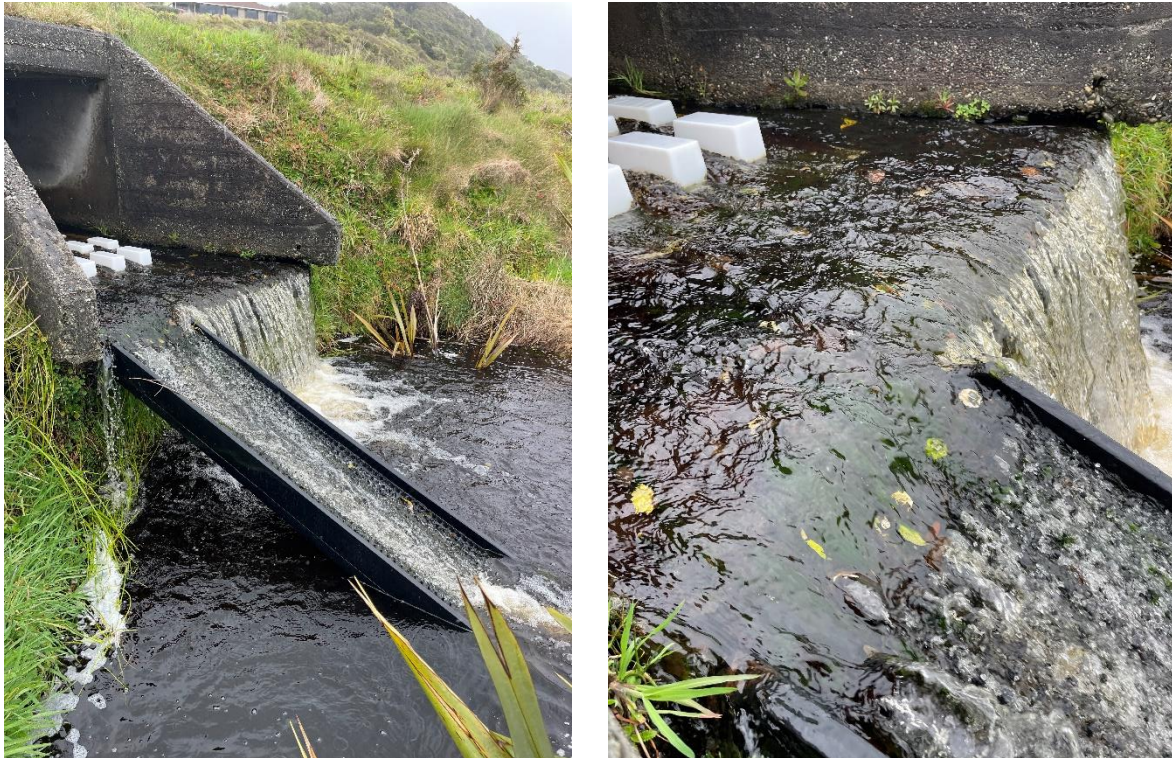
Figure 5-24: Artificial substrate ramp installed at a perched culvert on the West Coast. There are multiple ways this installation could be improved. Left: The entrance to the ramp extends past the upstream limit of migration and the ramp is too steep (~35°). The end of the culvert apron is also left unbaffled, which creates a high velocity impediment for any fish able to surmount the ramp. Right: Close-up of the ramp crest showing a high velocity barrier created by the smooth flexible crest used for ramp attachment and the lack of baffling at the crest. Note: this substrate is not Miradrain™ (see Figure 5-20 & Figure 5-21). Photos: Cindy Baker.
