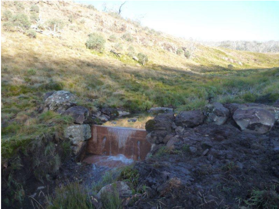
Figure 6-8: Example of a full exclusion barrier protecting a non-migratory galaxiid, Shaw galaxias, in Australia. The objective was to prevent trout accessing a key galaxias in Australia. Key features of the barrier were the height (1.3 m), shallow downstream zone to prevent trout access, infilling the upstream pool to provide stability for the barrier and prevent habitat for trout to jump into and placing large boulders on floodplain to direct overflow into the middle of the channel. Photo credit: Tarmo Raadik.
