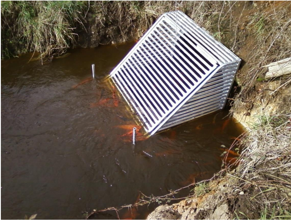
Figure 6-7: One-way gate fitted to Lake Ohinewai outlet drain, Waikato. The gate is designed to prevent adult koi carp from accessing the lake, while still providing small and other fish access to and from the lake. Credit: Adam Daniel.
