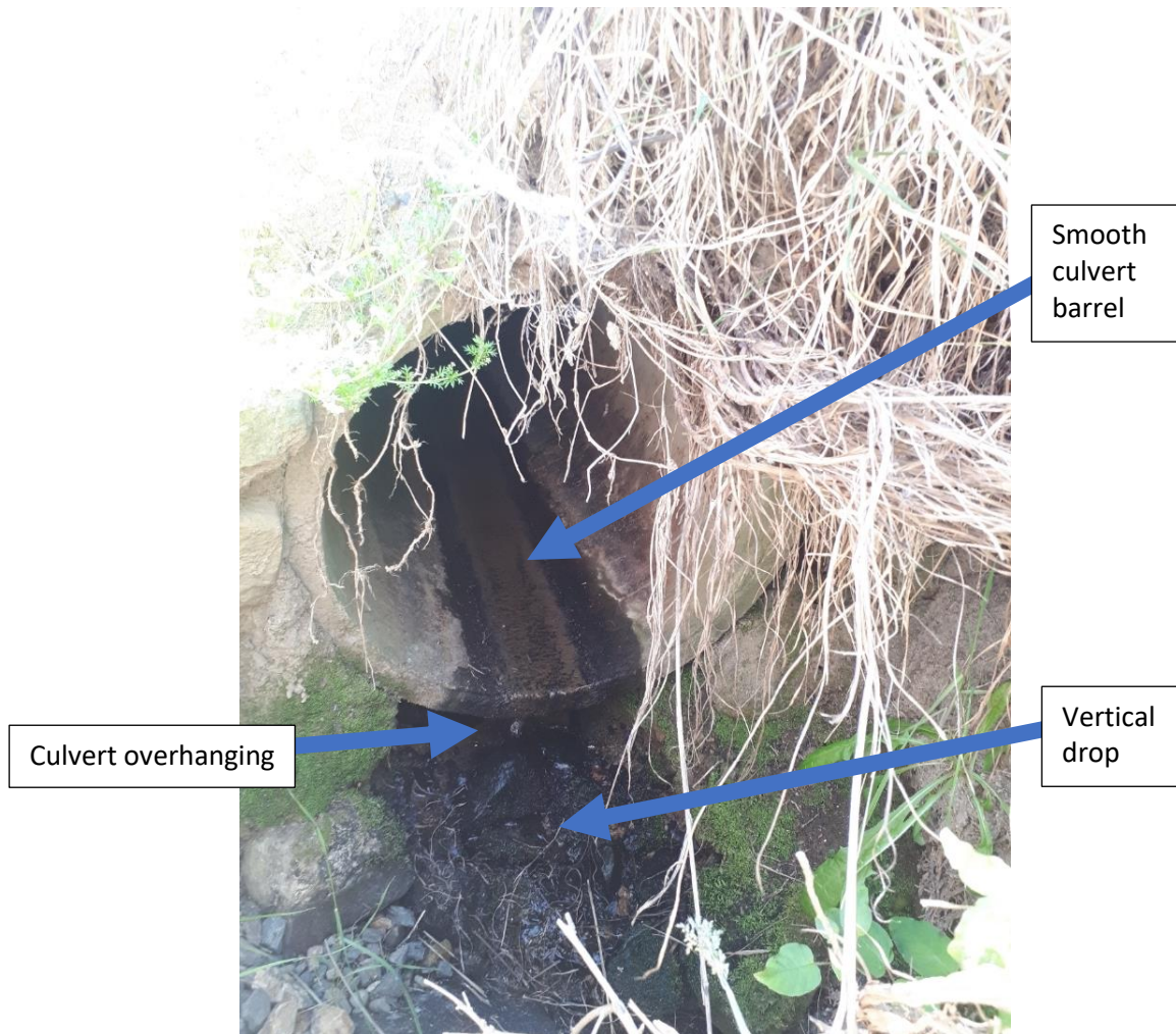
Figure E-15: Fish passage will be impeded by the fall height and undercut at the culvert outlet. The smooth culvert barrel will also lead to higher water velocities and limit fish movements under higher flows. Credit: Megan Brown.
