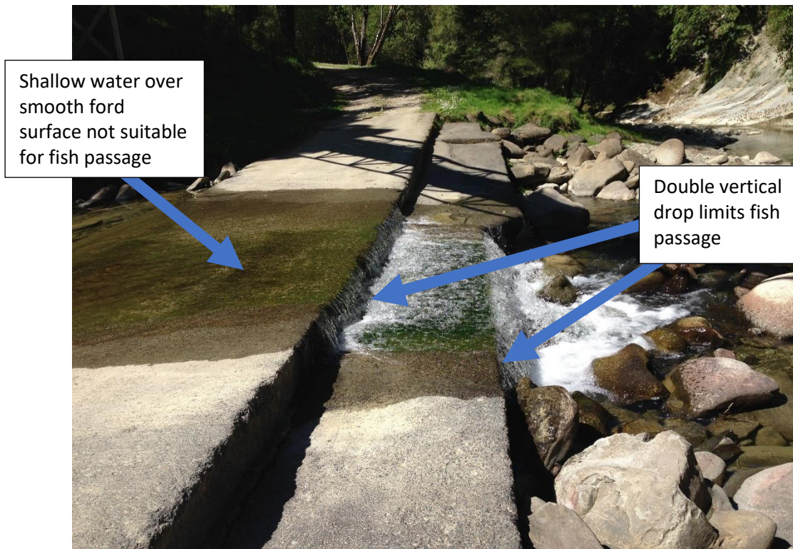
Figure E-20: Example of a ford from the Te Arai River. The fall height at the two steps on the downstream side of the ford makes a complete barrier to swimming fish species. Passage for climbing fish will be impeded by the sharp corners on the steps and shallow water across the ford, but some may access upstream habitats by taking advantage of the wetted margins to climb. Credit: Paul Franklin.
