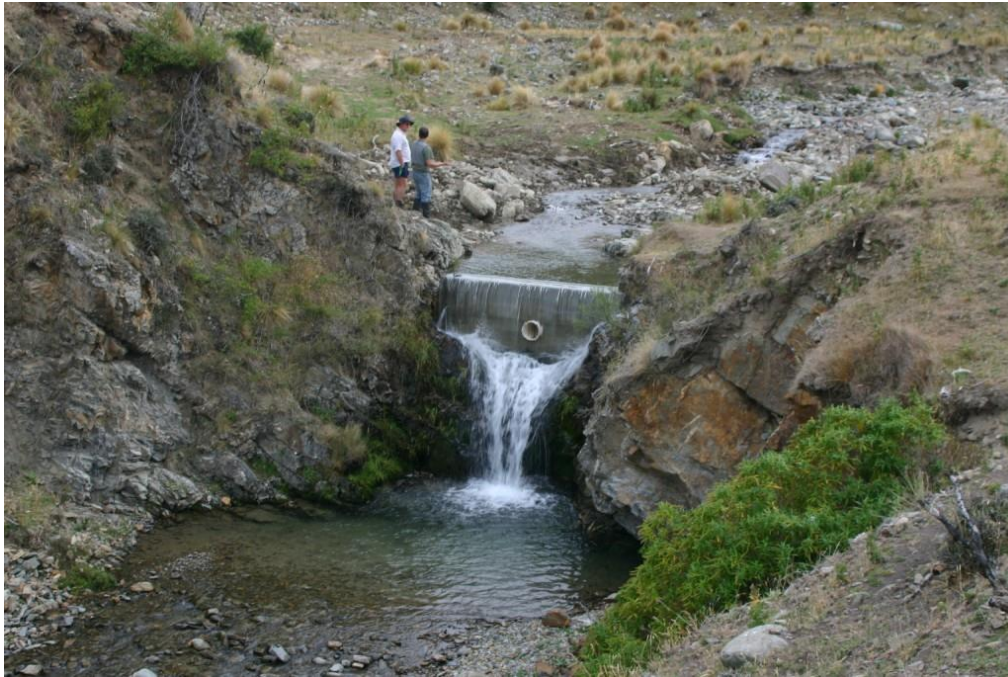
Figure 6-1: Swinburn Creek barrier in Otago. A built barrier has been installed onto a natural waterfall to protect Central Otago roundhead galaxias populations, after brown trout gained access upstream when stream conditions changed. Credit: Daniel Jack (DOC).
