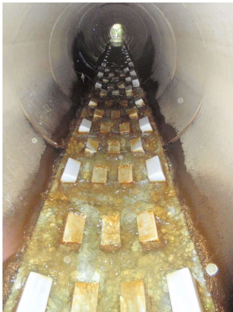
Figure 5-7: Spoiler baffle sheets installed inside a culvert.
