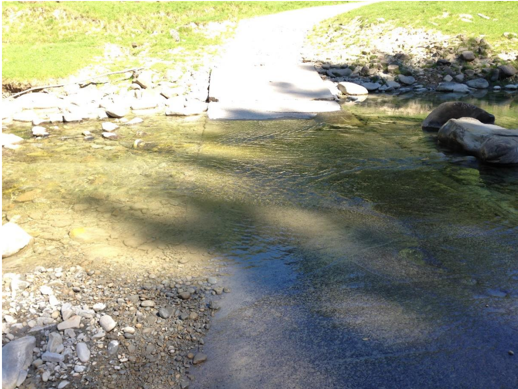
Figure 4-15: Low profile ford crossing.
