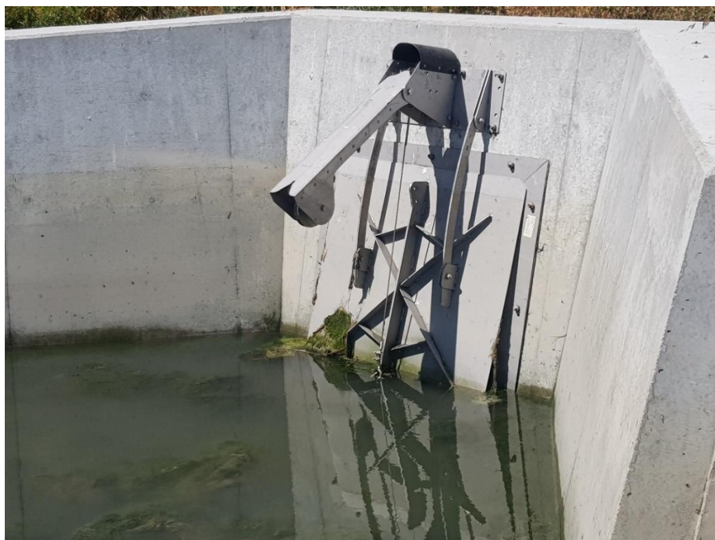
Figure 4-19: Example of a self-regulating tide gate installed in Canterbury. The counter weight system holds the tide gate open for longer on the incoming tide. The system can be calibrated to manage the magnitude and duration of the opening to best coincide with critical migration periods, e.g., the incoming tide for whitebait and eelers.
