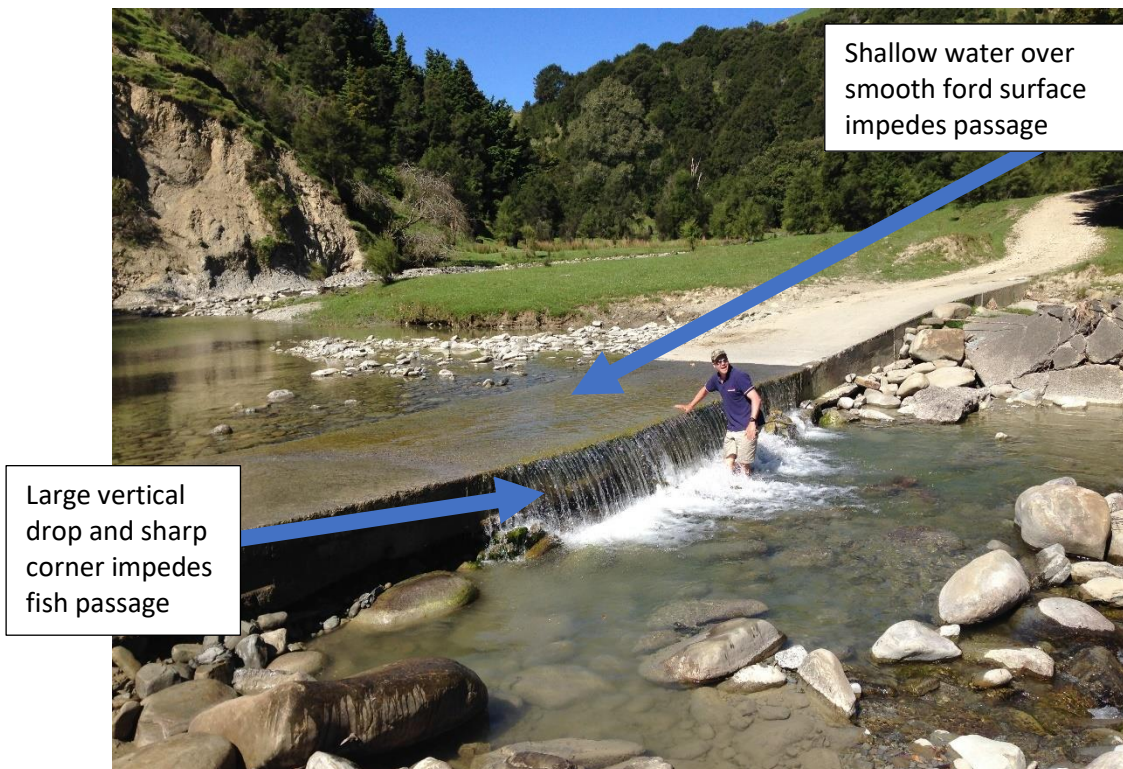
Figure E-21: The fall height on this ford on the Te Arai River is a significant impediment to the upstream passage of fish. Credit: Paul Franklin.
