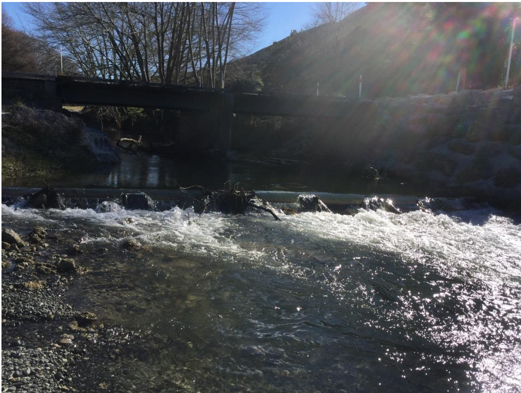
Figure 3-3: Rock-ramp installed in the Aropaoanui River, before (top) and after (bottom) an 80 \text{ m}^3 \text{ s}^{-1} flood. The rock-ramp was installed to overcome the barrier created by a historic weir (visible in the bottom picture after the rock-ramp was washed away). However, the rock-ramp design was insufficient to withstand the flood meaning that reconstruction is required to restore fish passage at the weir. Credit: Andy Hicks.
