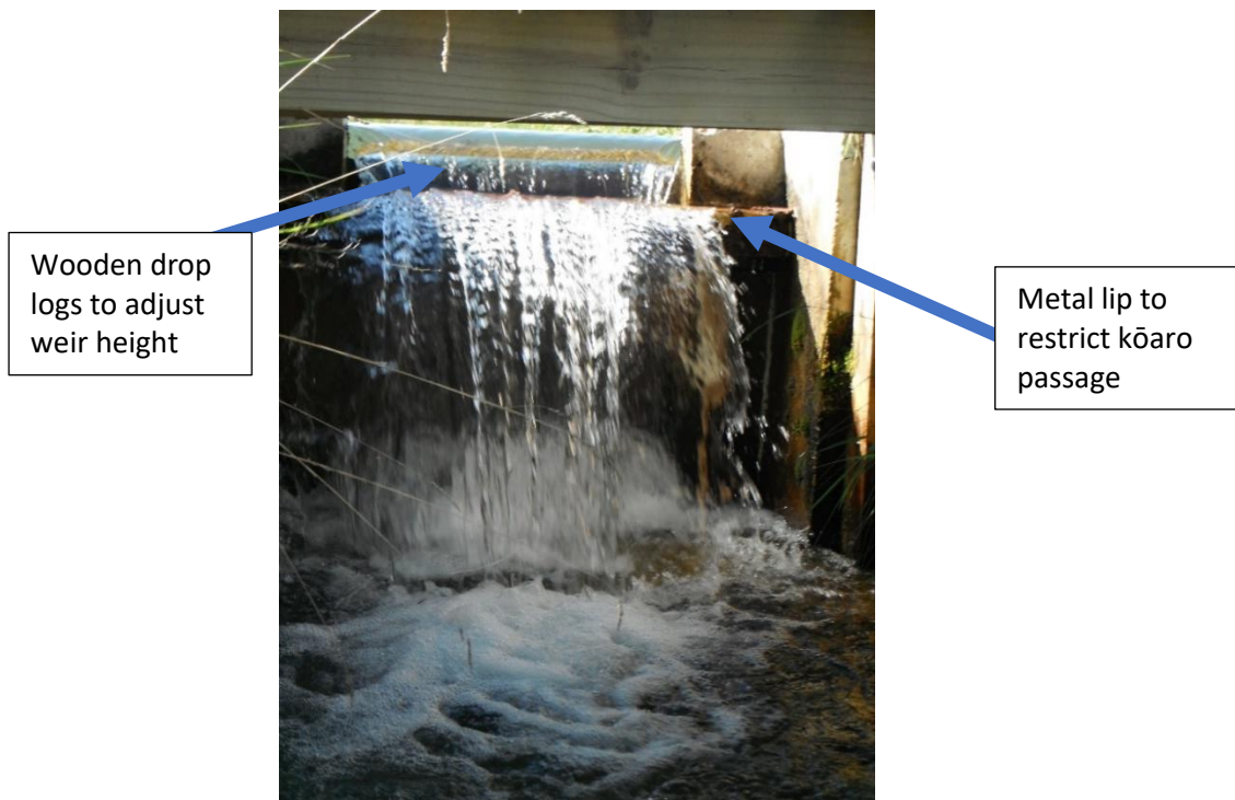
Figure 6-5: Built barrier installed in an unnamed spring of the Fraser River. The objective of this built barrier was to prevent trout and kōaro accessing a key lowland longjaw galaxias and bignose galaxias stronghold in the MacKenzie Basin, Canterbury. Key features of the barrier were the height to prevent trout access, the metal lip to prevent kōaro passage, and the wooden drop logs to allow for flushing of flows and maintenance of flows and habitat upstream. Credit: Sjaan Bowie (DOC).
