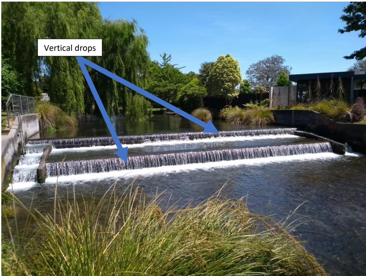
Figure E-13: Example of a weir in central Christchurch. Fish passage will be impeded by the fall height of the steps in the weir and the salmonid fish passes. Credit: Megan Brown.
