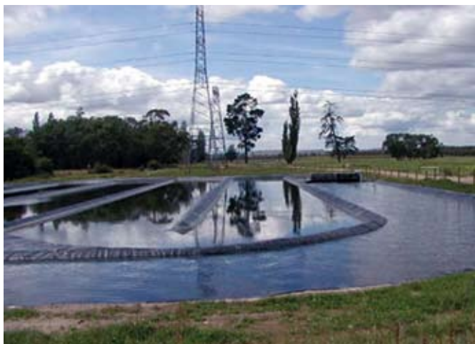
Aerobic pond designed for growing algal biomass and scrubbing CO 2 .
