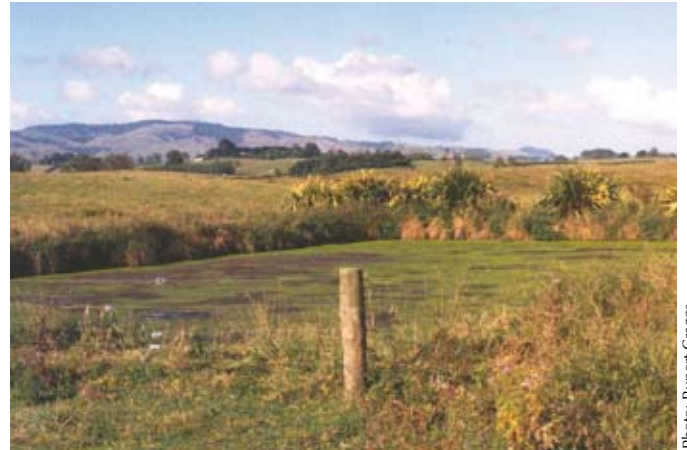
Conventional anaerobic pond used for treatment of dairy farm wastewater.
