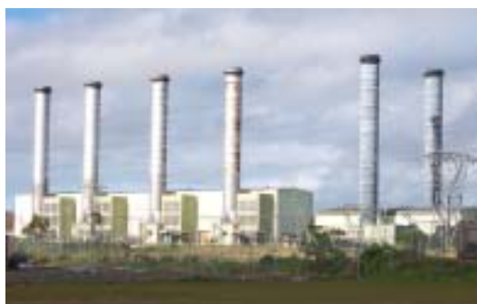
Power generation in south Auckland
