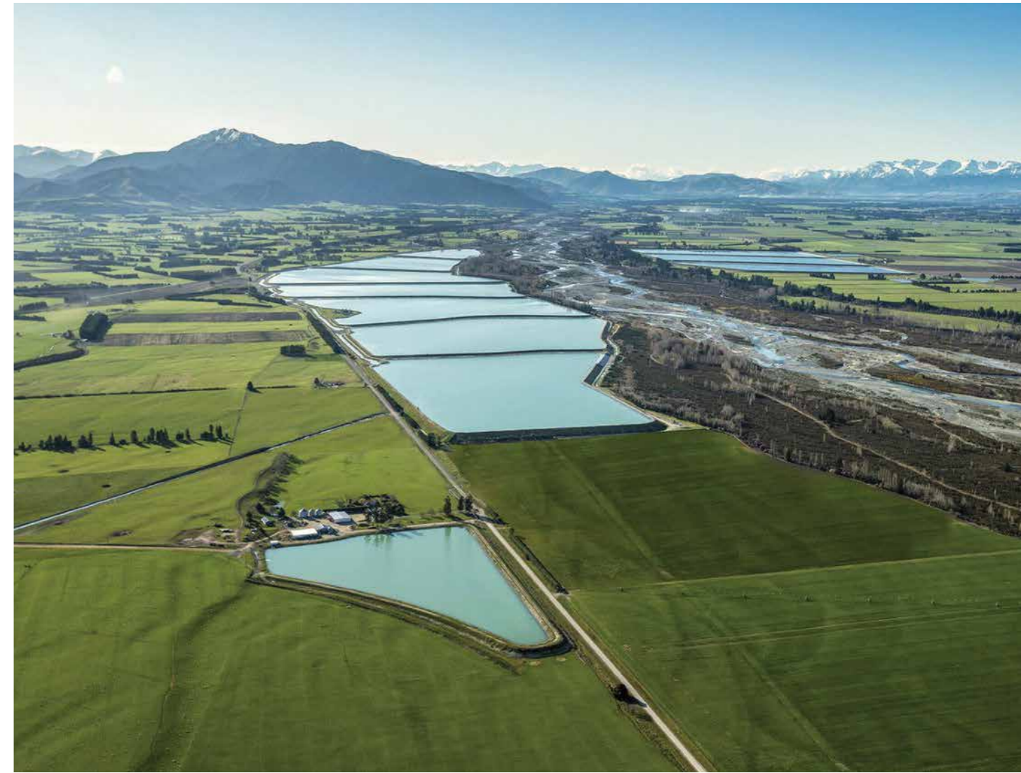
NIWA-supplied automation controls water in and out of the Rangitata South Irrigation Scheme ponds. The ponds are about 1km across at the widest point and 5km long. [Rooney Earthmoving]
