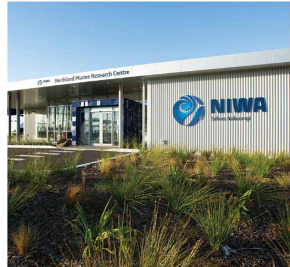
The new administration building at NIWA’s Northland Marine Research Centre has transformed the facilities at the Centre. The experimental, commercial-scale recirculating aquaculture system is being constructed on the left of the new building. [Cato Brand Partners]
