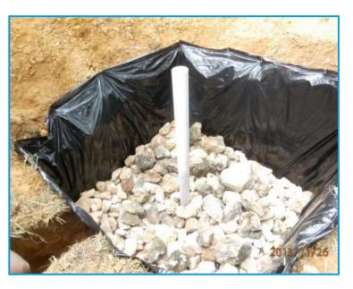
Figure 2. Soak pit under construction.
