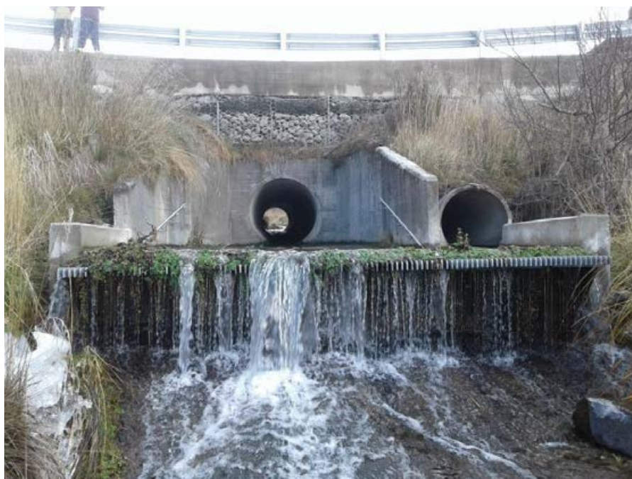
Figure 6-7: An example of an anti-jump screen/ grill that could be added to a barrier to prevent trout access. Photo credit: Sjaan Bowie.
