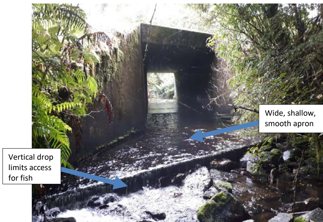
Figure B-17: Fish movements will be impeded by the fall at the downstream end of the apron and shallow water on the apron. Photo credit: Sam Ammon.
