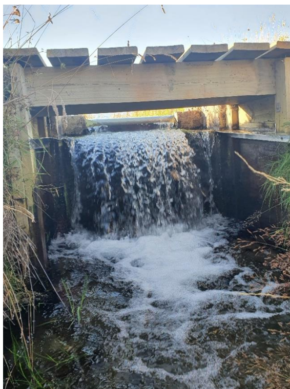
Figure 6-6: Exclusion barrier installed in an unnamed spring of the Fraser River. The objective was to prevent trout and kōaro accessing a key lowland longjaw galaxias and bignose galaxias stronghold in the MacKenzie Basin, Canterbury. Key features of the barrier were the height (0.83 m) and shallow downstream zone (concrete splash pad) to prevent trout access, the metal lip (300 mm wide at barrier face, 100 mm on concrete sides, 150 mm on wooden sides of bridge) to prevent kōaro passage (seems to be unsuccessful), and the wooden drop logs to allow for flushing of flows and maintenance of flows and habitat upstream. Photo credit: Sjaan Bowie (DOC).
