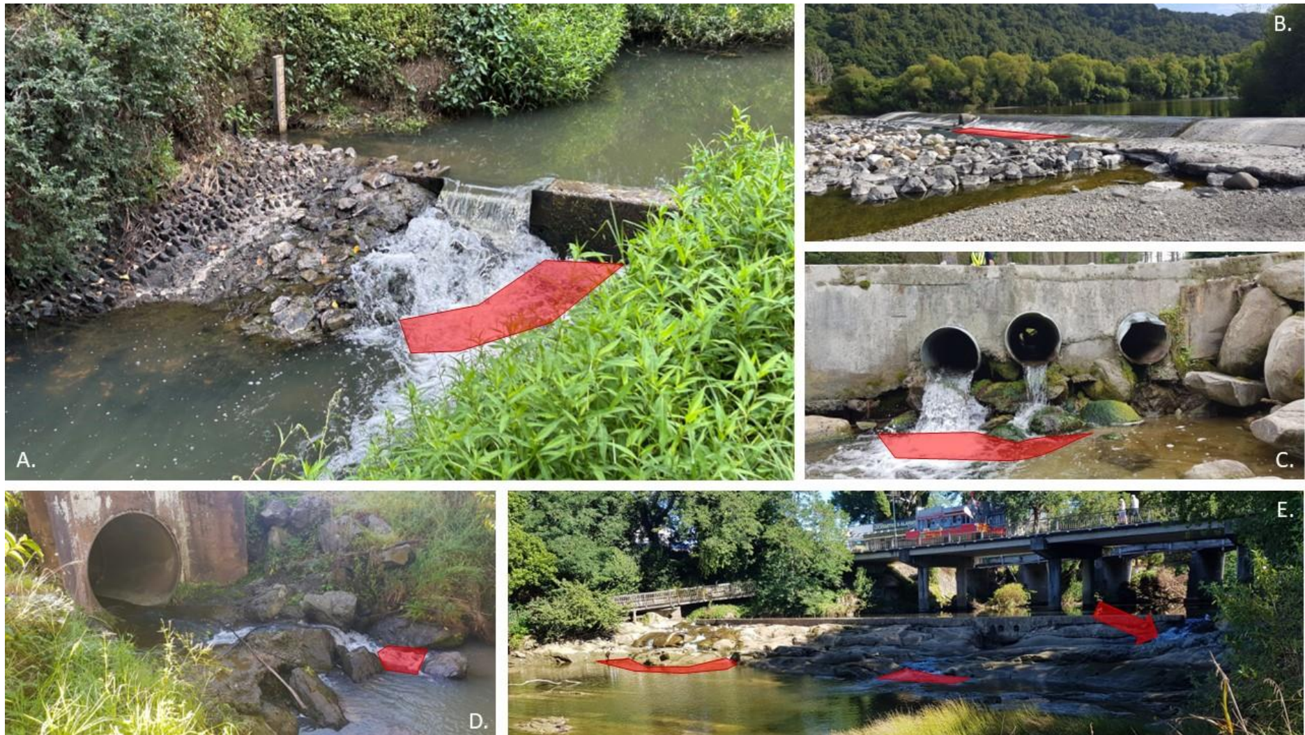
Figure 5-12: Locating the upstream limit of migration (area shaded in red). The upstream limit of migration is the furthest point upstream that fish can move to. The red areas show the upstream limit of location for structures A-E at the time the picture was taken. Note that site E is tidal and the upstream limit of migration moves from the shaded areas to the location indicated by the arrow at high tide.
