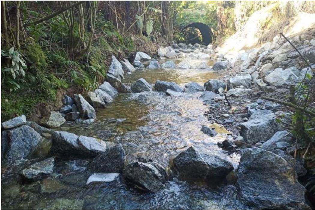
Figure 5-9: Example of a full-width rock ramp fishway in Mill Creek, West Coast. Photo credit: Koen Beets.
