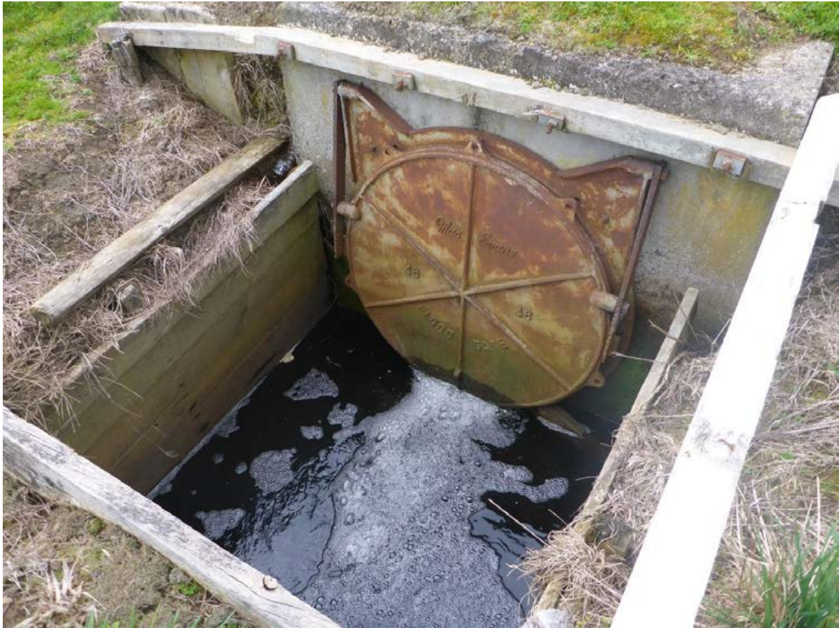
Figure B-8: An example of a tide gate from the Waikato River catchment. Photo credit: Rimutere Wharakura.
