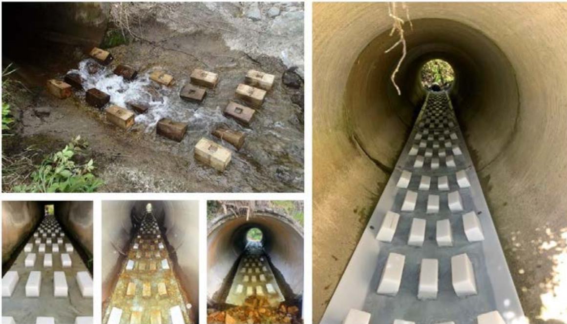
Figure J-2: Examples of spoiler baffles.
