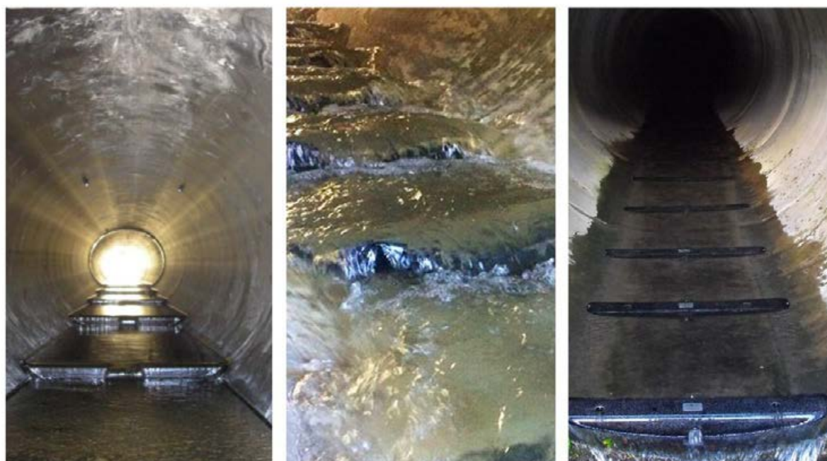
Figure J-1: Examples of weir style baffles including slotted baffles (Left), flexi-baffles (Centre) and standard weir baffles (Right).
