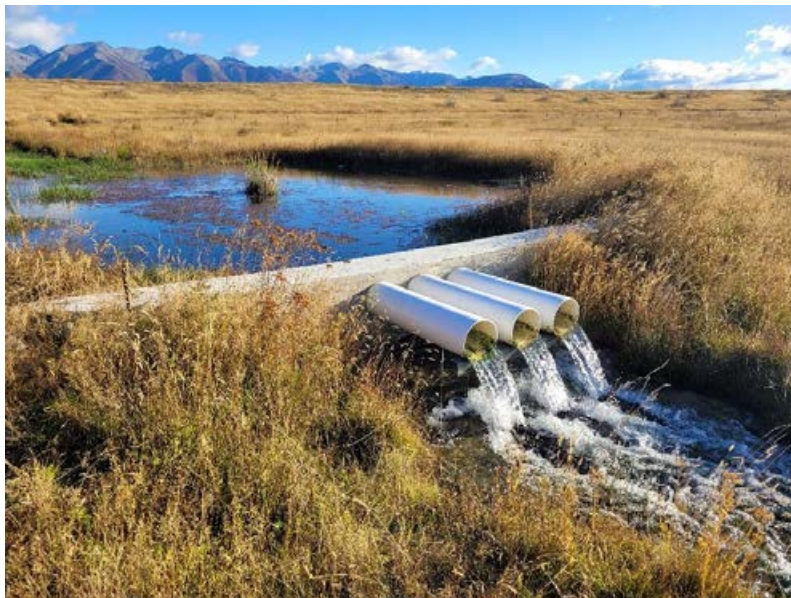
Figure 6-5: Low-head exclusion barrier installed in an unnamed spring, Waterwheel Wetland, Canterbury. The objective was to prevent trout and kōaro accessing a key bignose galaxias stronghold in the MacKenzie Basin, Canterbury. Key features of the barrier were the height (0.31 m fall from end of pipe to concrete splash pad) and downstream shallow zone (1.95 m of concrete splash pad below the pipes) to prevent trout access and the 0.62 m height and dry concrete face of the wall above the concrete pad to prevent kōaro and trout passage. Photo credit: Sjaan Bowie.
