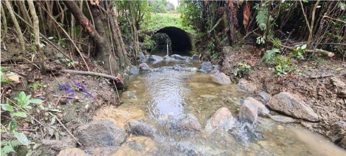
Figure 5-14: Example of a newly constructed full width rock ramp fishway in Mill Creek, West Coast. Photo credit: Tim Marsden, Australasian Fish Passage Services.
