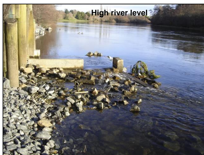
Figure 5-16: Example of a formal concrete rock ramp below a culvert that is oriented perpendicular to the downstream water body. A receiving pool has been added to the base of the culvert with the ramp directed downstream along the river margin. This provides the foundations for a low gradient sloping ramp. The orientation along the river margin increases the attraction efficacy of the ramp and allows flood flows to be spilled over the receiving pool, perpendicular to the river flow.
