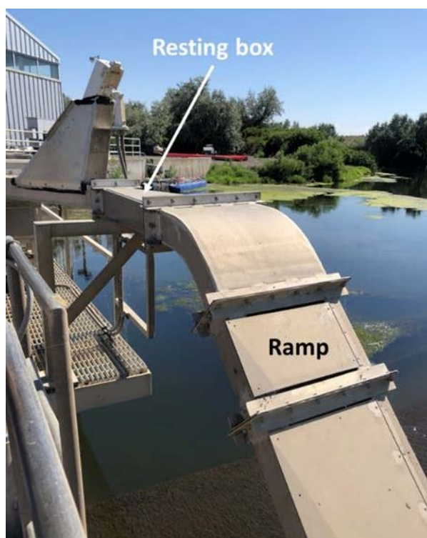
Figure 7-12: Example of a resting box in a LPS designed for Pacific lamprey passage at Three Miles Falls Dam, Umatilla River, Oregon. Photo credit: Cindy Baker.
