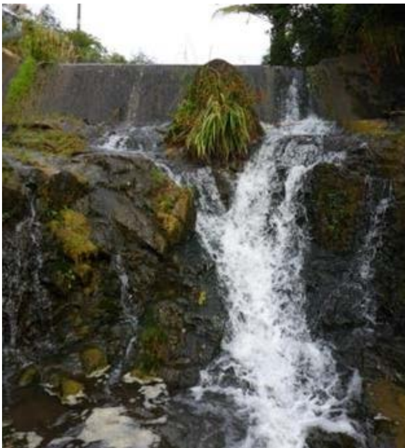
Figure 6-14: A weir built on top of a natural waterfall in Waitawhara Stream, Waikato. Although not designed as a selective barrier, the weir and waterfall prevent koi/amur carp, goldfish, perch, rudd, gambusia and catfish from accessing headwater habitats while allowing the passage of banded and giant kōkopu and shortfin and longfin eels. Key features of the barrier include the roughness and wetted margins that desirable fish use to migrate, plus a rounded crest on the concrete weir. Photo credit: Cindy Baker.
