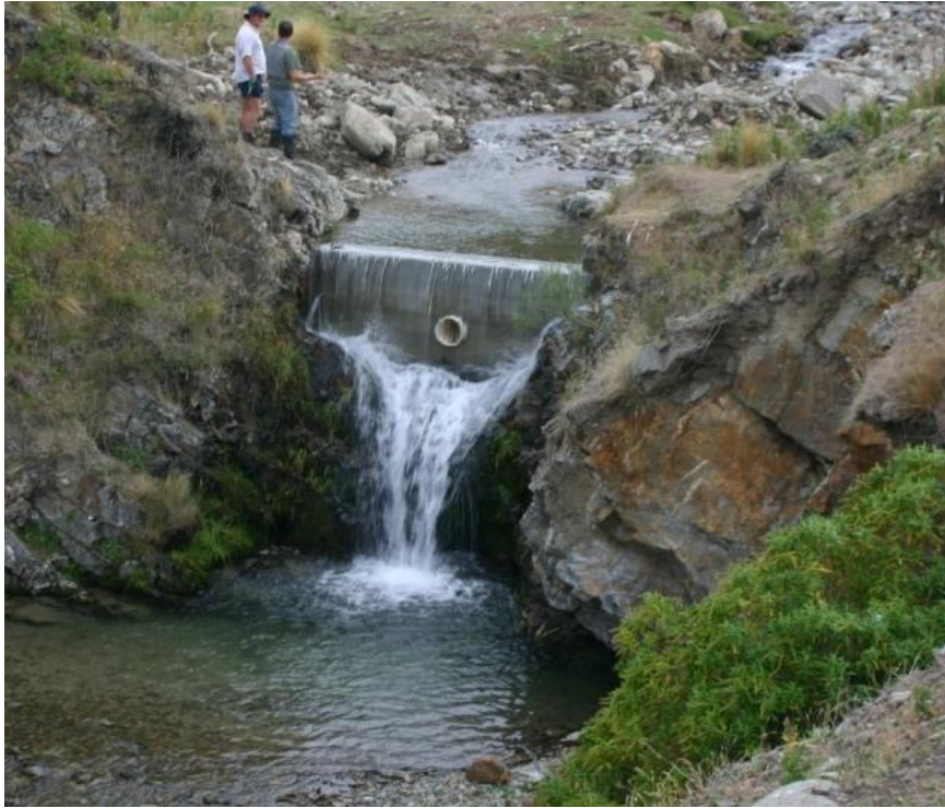
Figure 6-2: Swinburn Creek barrier in Otago. A high head exclusion barrier has been installed onto a natural waterfall to protect the Central Otago roundhead galaxias population, after brown trout gained access upstream when stream conditions changed. Key features of the barrier are the height to prevent trout access. Photo credit: Daniel Jack.
