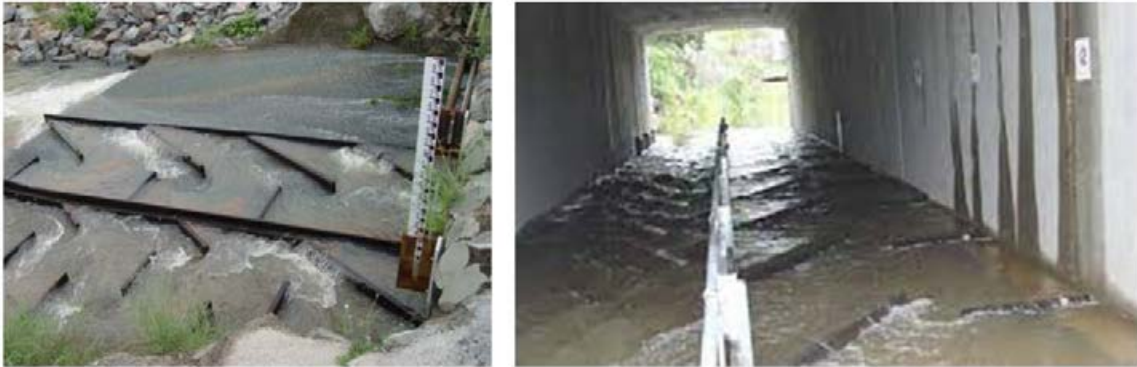
Figure J-4: Examples of offset baffles. Source: Kapitze (2010).
