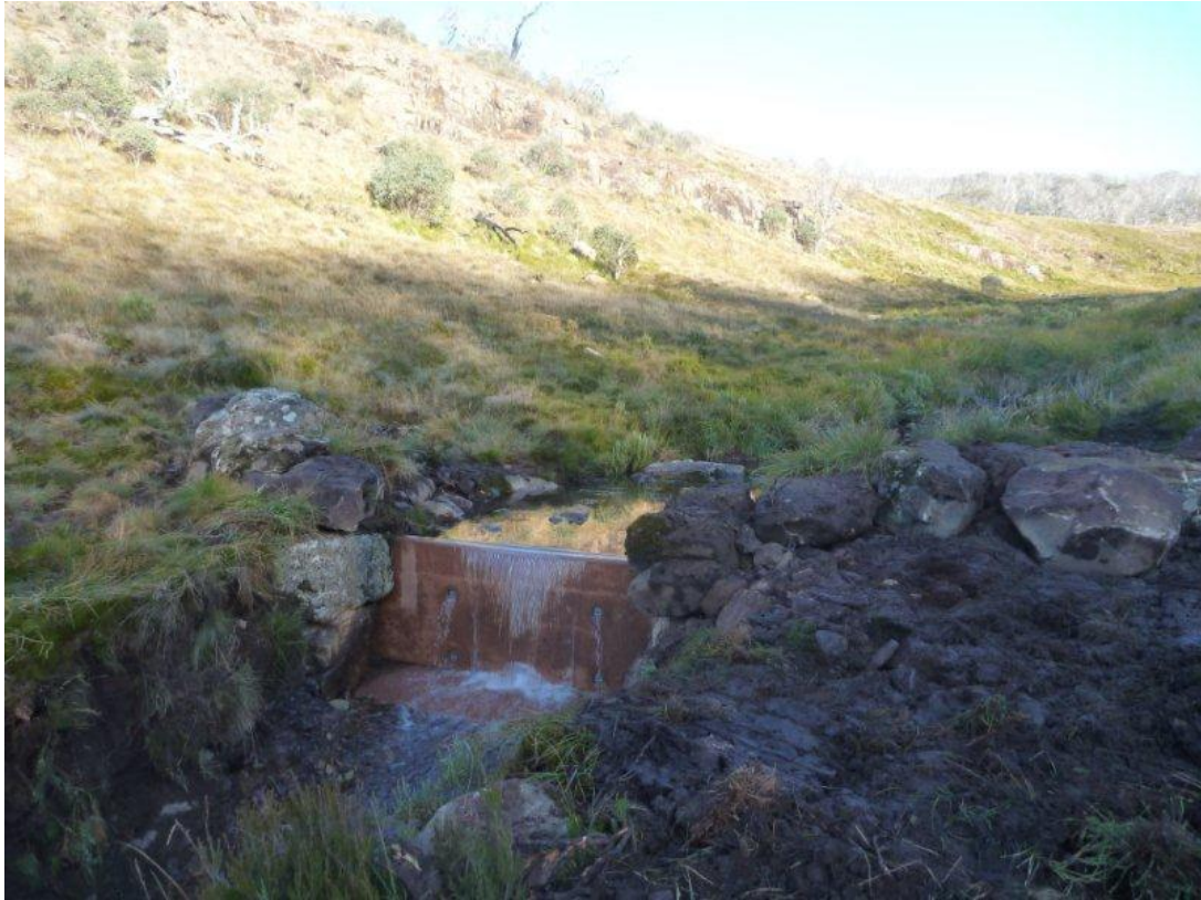
Figure 6-8: Example of a full exclusion barrier protecting a non-migratory galaxiid, Shaw galaxias, in Australia. The objective was to prevent trout accessing a key galaxias in Australia. Key features of the barrier were the height (1.3 m), shallow downstream zone to prevent trout access, infilling the upstream pool to provide stability for the barrier and prevent habitat for trout to jump into and placing large boulders on floodplain to direct overflow into the middle of the channel. Photo credit: Tarmo Raadik.
