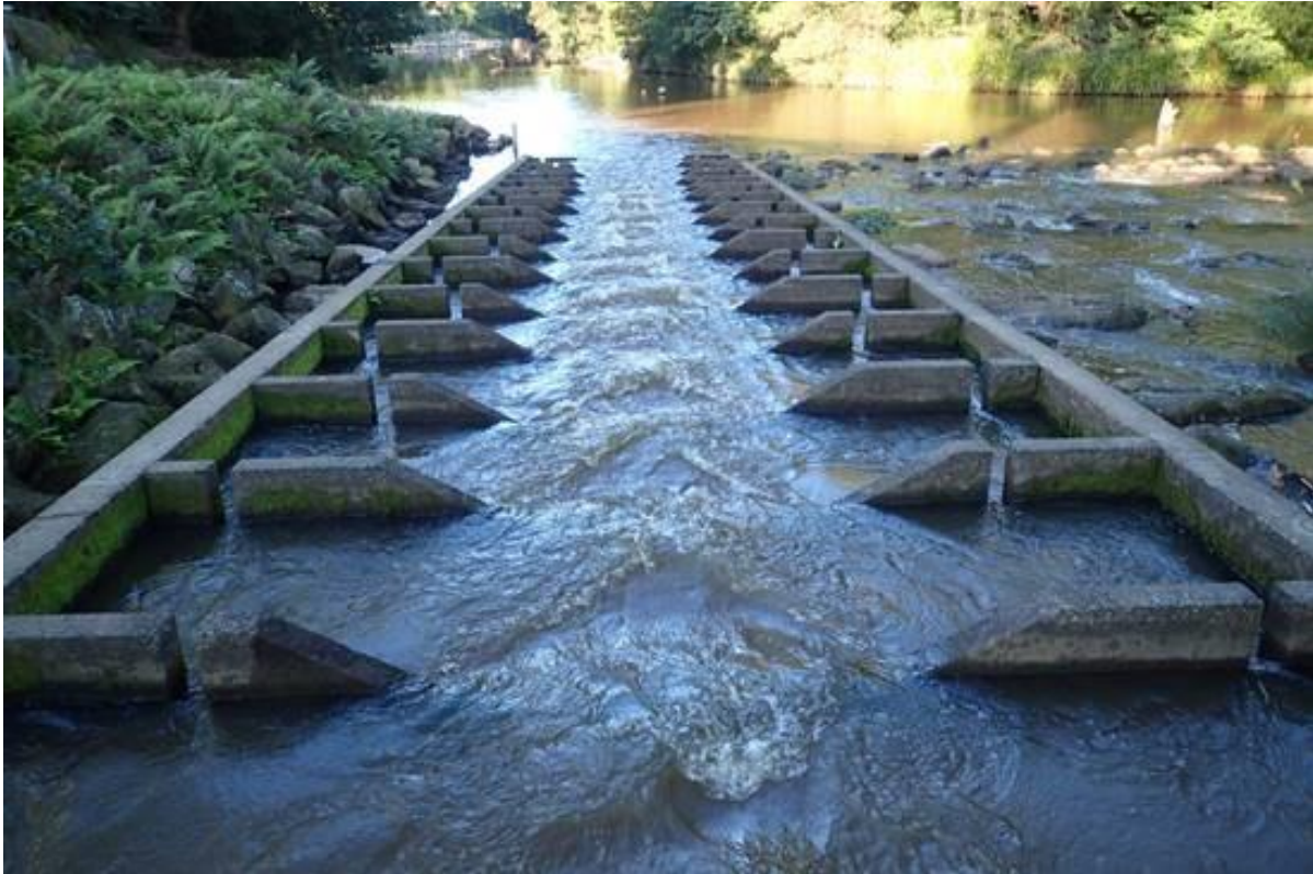
Figure 7-22: Trapezoidal fishway, Wyong River, New South Wales. Photo credit: Tim Marsden.
