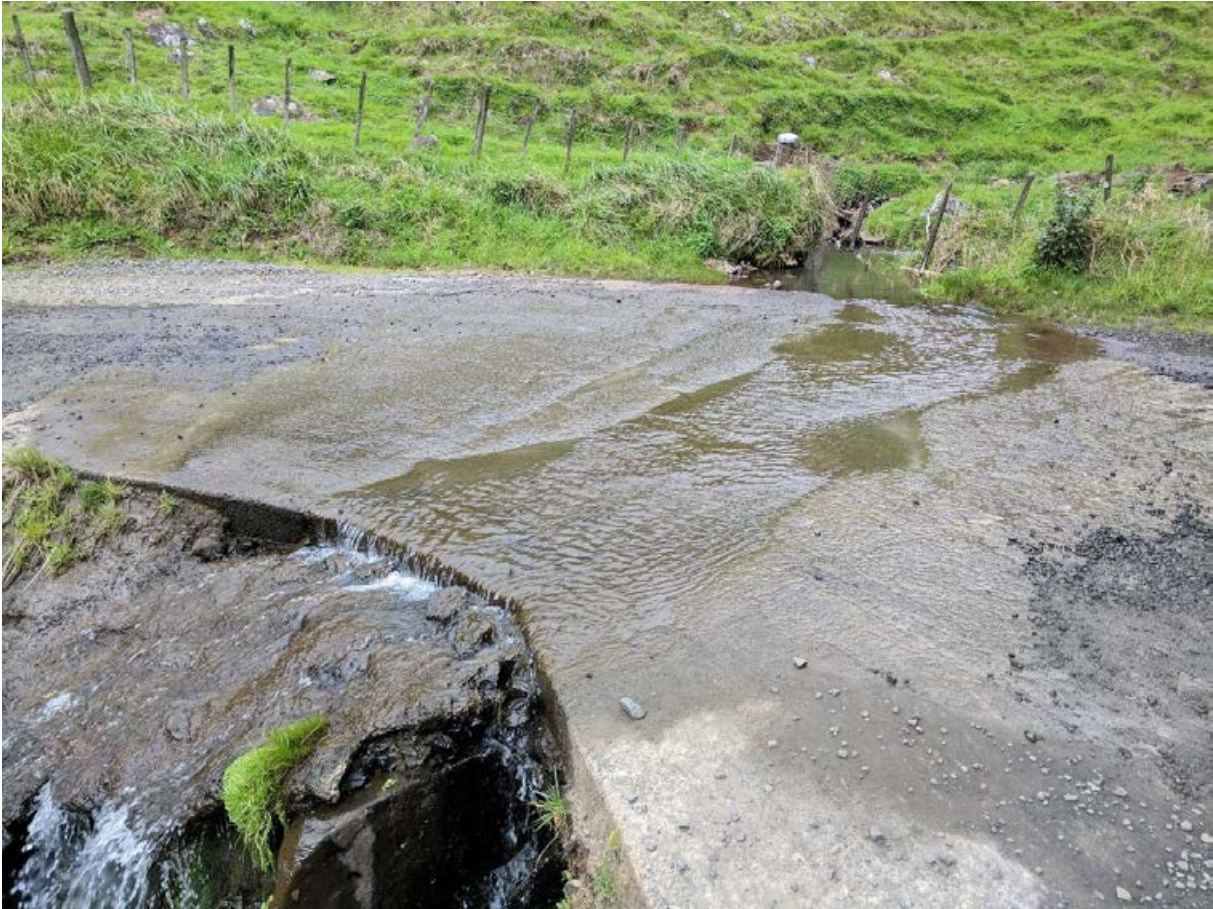
Figure B-6: Example of shallow water that can act as a barrier to movement for fish. Photo credit: Eleanor Gee.
