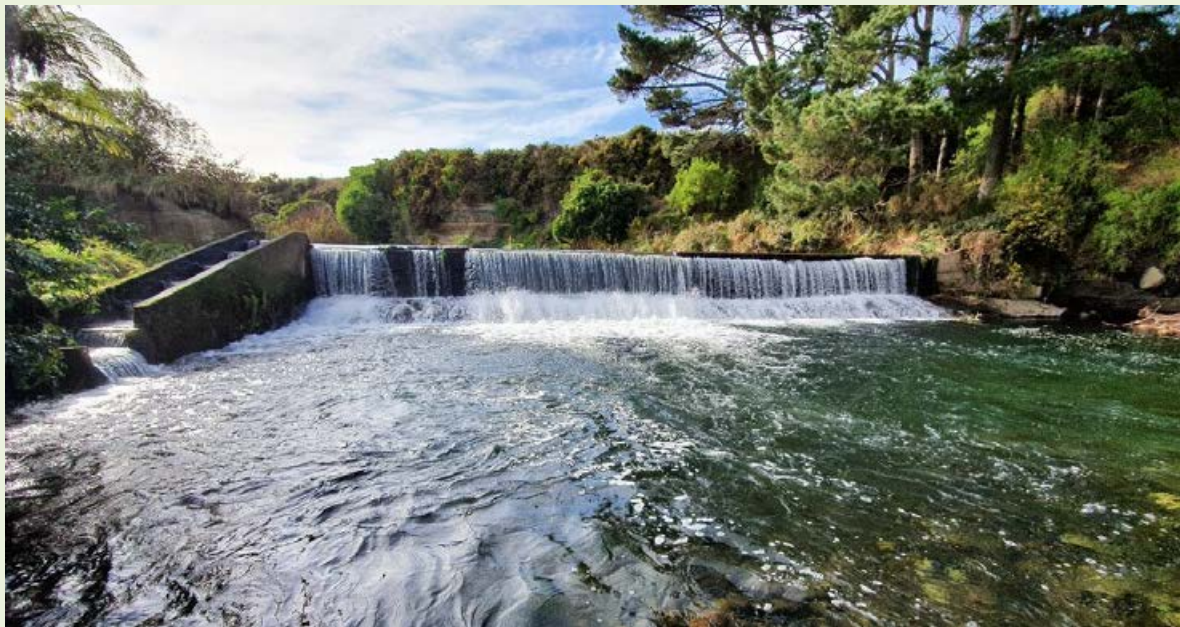
Figure 5-4: Kaūpokonui Stream weir prior to removal in 2021. Photo credit: Te Korowai o Ngāruahine.
