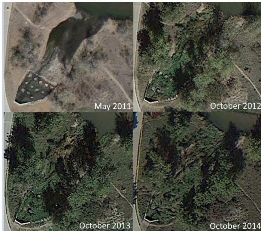
Figure G-3: Vegetation growth as part of soil rip-rap at stormwater outfall over four years following construction.
