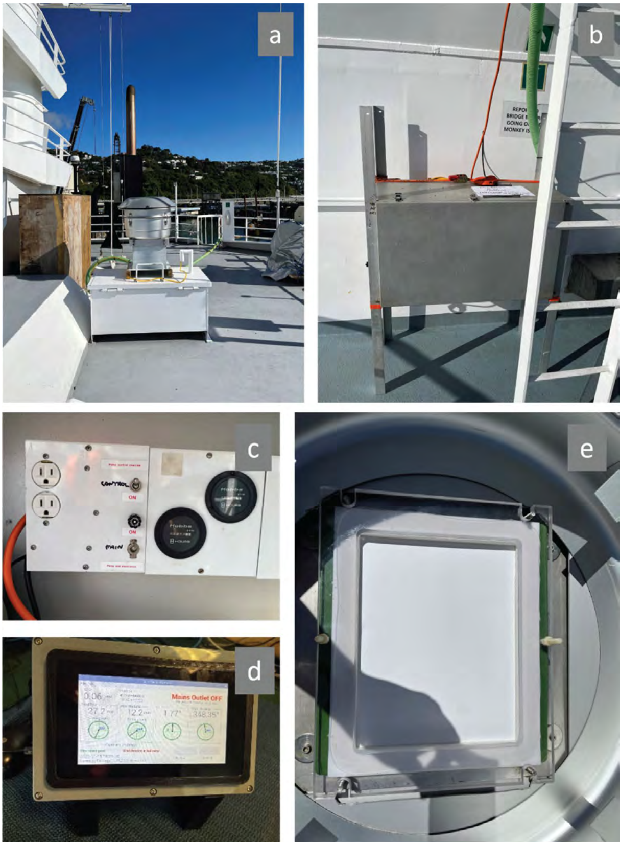
Figure 27: High-volume aerosol sampler (hi-vol). a) Installation location on the monkey island. The hinges can be taken off to allow the top of the hi-vol to be removed and a filter to be installed. The green hose follows along the ladder to the Monkey Island. b) The green hose attaches to the pump system on the mezzanine floor. c) The pump control panel, with control set to automatic to give control to the wind sector control panel. d) Wind sector control panel determines whether the wind is flowing from the right direction and subsequently turns the pump on. e) Example of a quartz microfibre (QMA) filter mounted in the hi-vol cassette.
