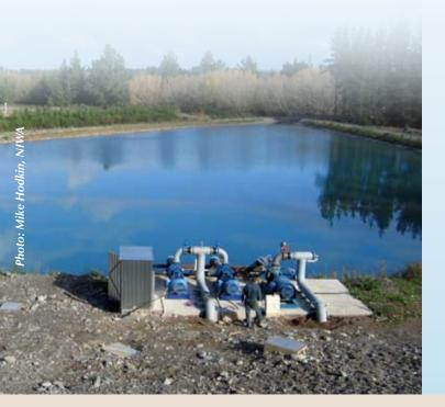
In the most recent project, Instrument Systems and Environmental Consultancy Services Ltd built, installed, and commissioned a flow monitoring and control station on the Glenroy Irrigation Scheme. The Glenroy scheme, near Darfield, has resource consent to divert up to 3.5 cubic metres of water every second from the Rakaia River, and uses this to fill a large reservoir. Two dairying companies, Canterbury Grasslands Ltd and Lynton Dairy Ltd, use water from the scheme for irrigation.
