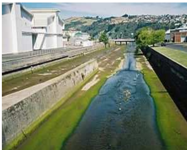
Looking downstream towards the outlet of the Leith to the harbour
