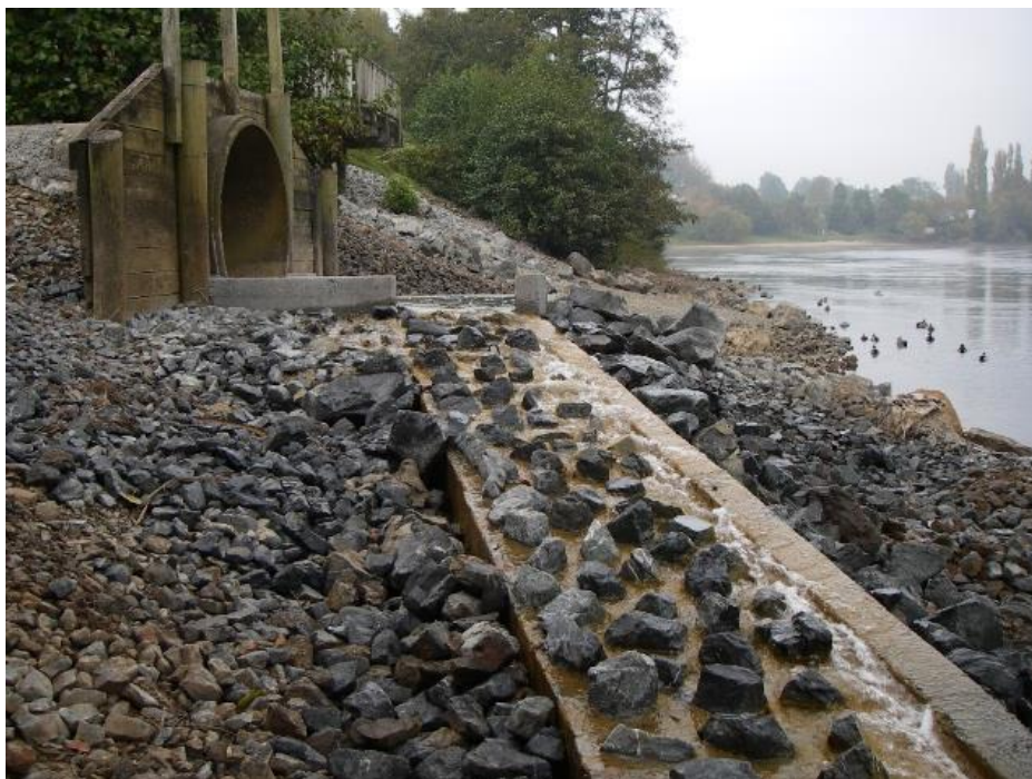
Figure E-2: Example of a fish ramp installed downstream of a culvert.
