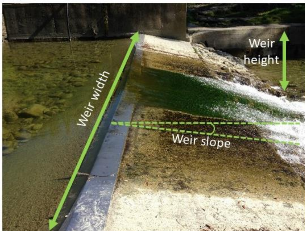
Figure D-3: Illustration of where to take key measurements for weirs.
